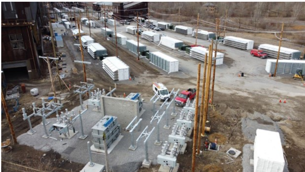
Construction underway at the Midland, PA site.
