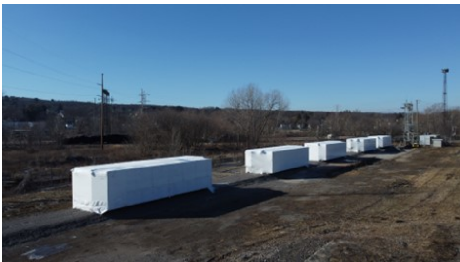
Aerial view of Sharon, Pennsylvania facility expansion
