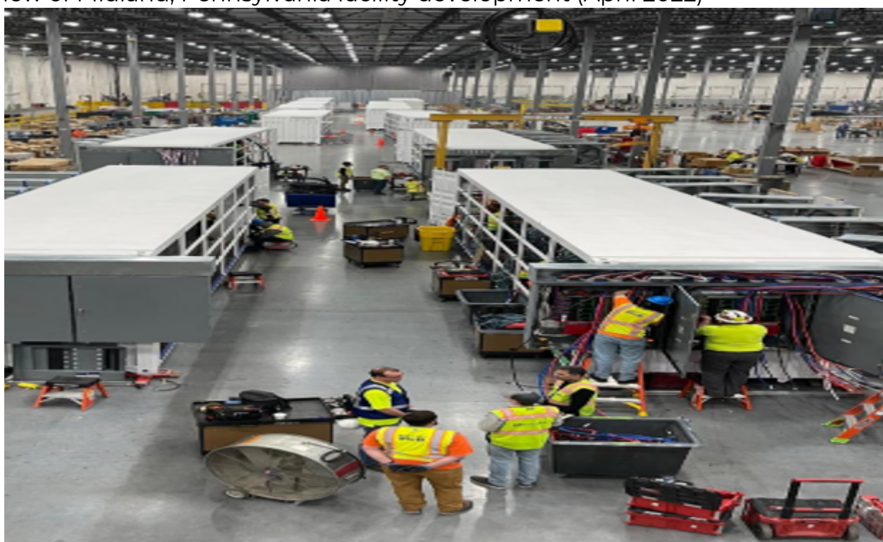
USA Modular Data Center (MDC) fabrication facility
